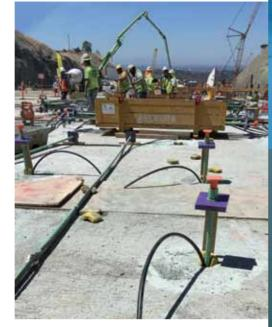
**ABOVE. PLANIGROUT** 755 was pumped in to fill the voids between the pieces of rebar and the outer wall of the core
